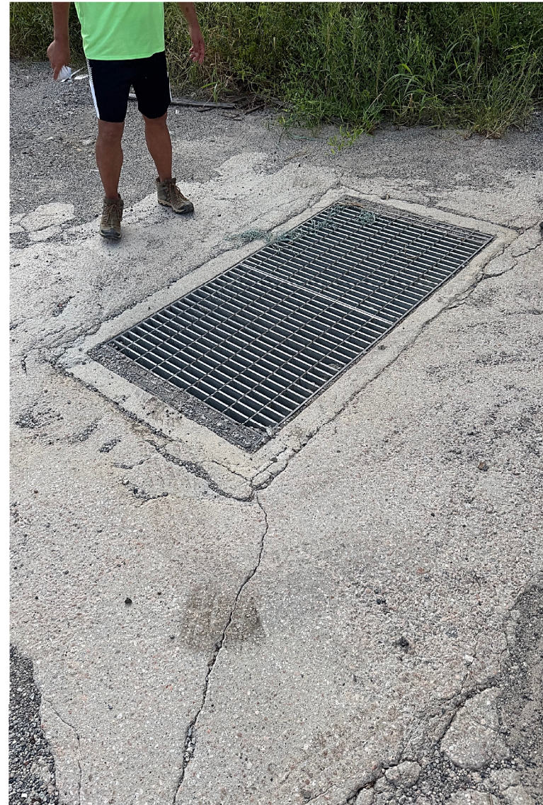
Photo 2 showing the last Manhole MH E
