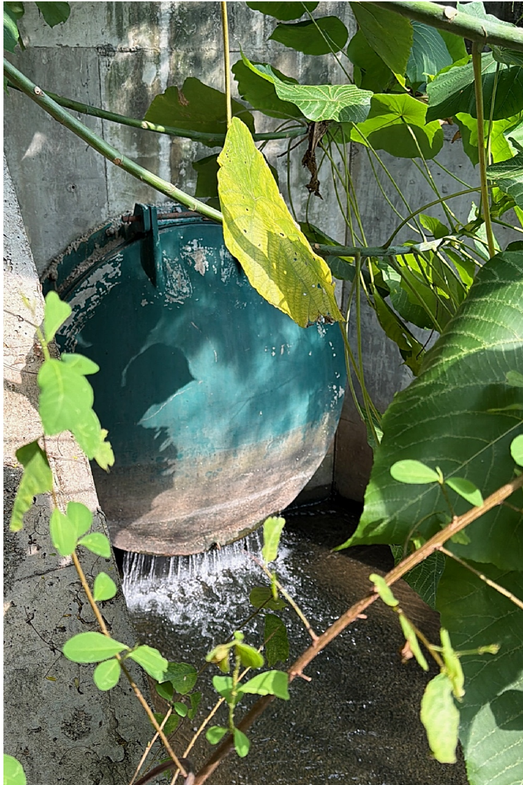
Photo 3 showing the Ultimate Outfall
